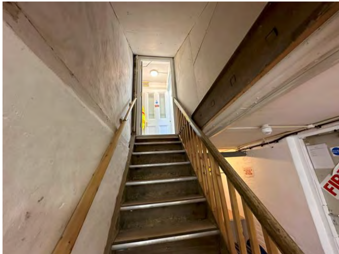
Staircase leading down to Basement
