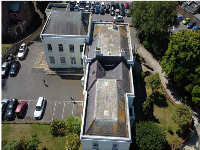
Drone image of a combination of roofs - facing South
