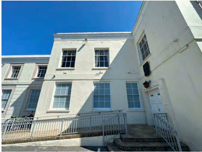
External Southern Elevation: ramped approach to New Millennium Chamber lobby
