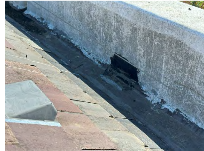
Liquid applied waterproof coating / repairs to back gutters behind parapet walls
