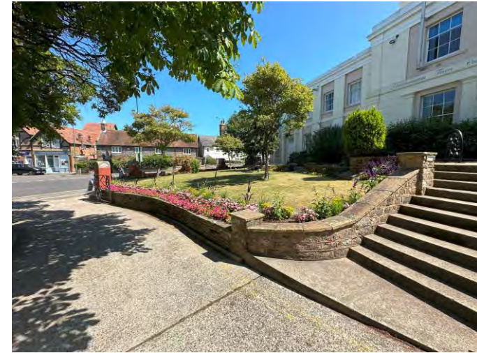
Concrete roadway, entrance steps and masonry retaining walls
