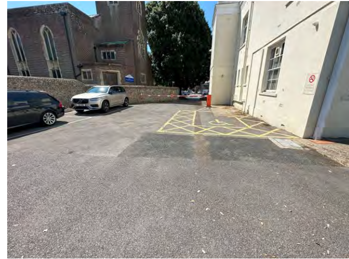
Rear car park – facing South
