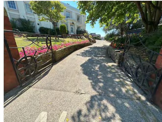
Entrance roadway, brick piers and metal gates
