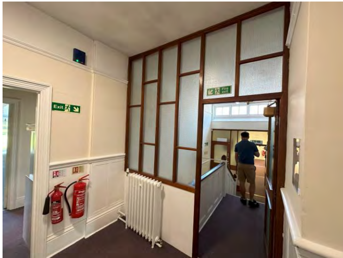
Glazed screen to stairwell lobby – Georgian wired glass
