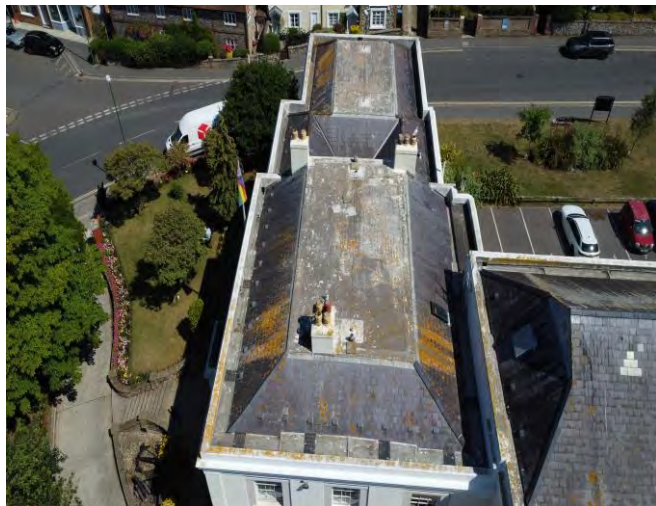
Drone image of the roofs – facing North
