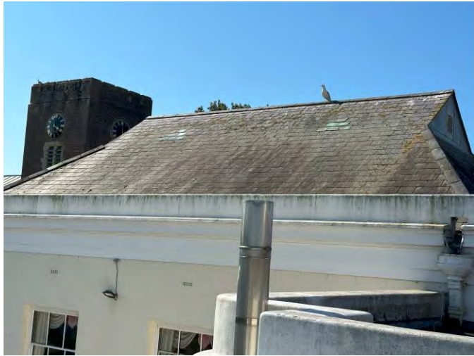
Roof above the New Millennium Chamber
