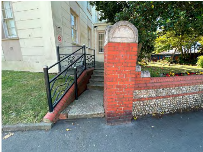
Concrete steps and handrail, masonry pier and flint infilled walls
