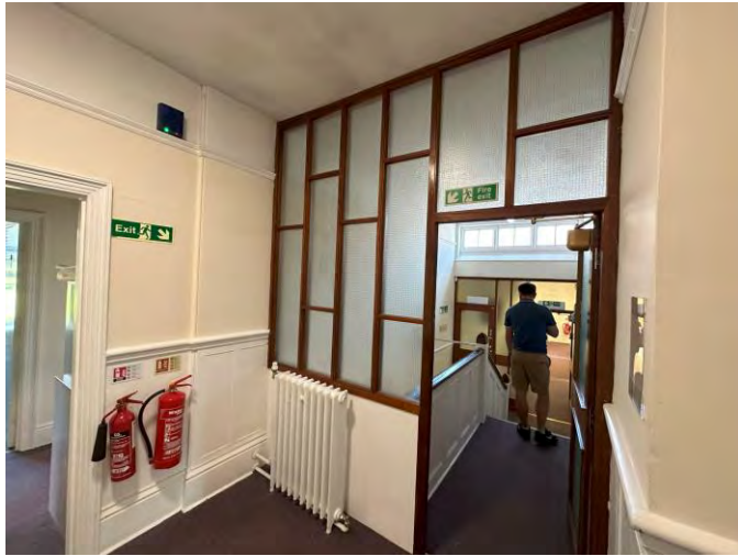
Corridor (112) and Stairwell
