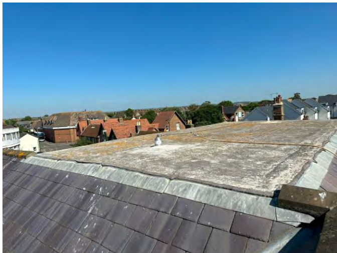
Mansard roof – asphalt roof covering
