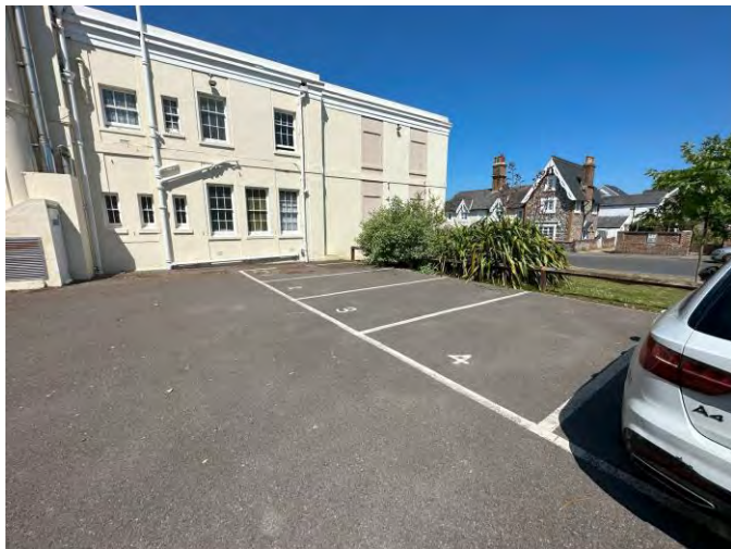
Car Park and road markings
